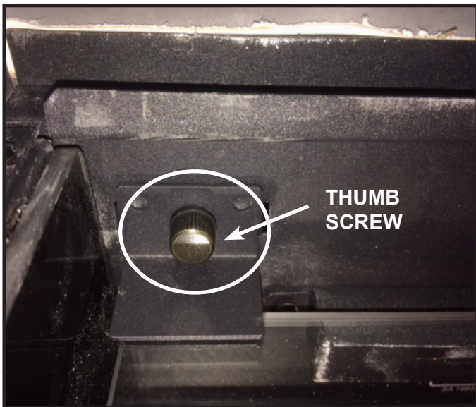
Figure 4.12 Glass Removal and Installation
