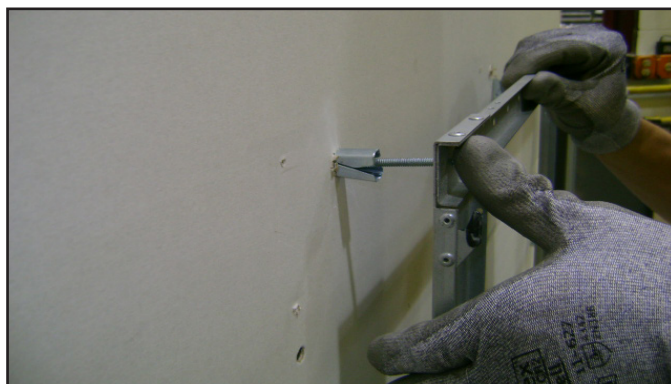
Figure 4.11 Installing Anchors in Hollow Wall
